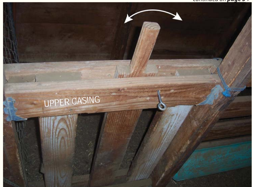
Vertical pivoting slat opens and closes against a stationary slat
